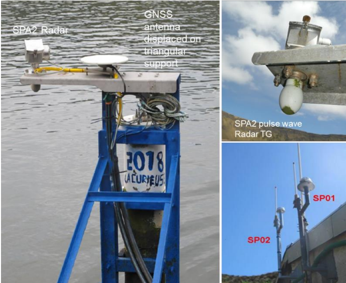
Figure 7 : Saint-Paul SPA1 and SPA2 stations in November 2018 upgraded with an open -air radar gauge (SPA2_RDR); SPA2 radar data are transmitted independently from SPA1 data by using two stations and ARGOS antennas (Adapted from Nivmer report photos)
